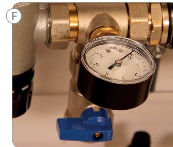
Connect the mains supply hose to the top flow bar red tap. Connect the drain off hose to the lower return bar blue tap, place the end of the drain hose into a bucket. Open both the red and blue drain taps, turn on the mains water supply to the fill hose.
