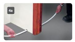
When floor heating pipes need to pass through walls, drill the holes before laying and fixing boards to prevent any damage to the boards. Protect and seal the pipe ends with tape. To prevent kinking, one person should feed the pipe through the hole whilst another draws the pipe through from the other side (4a).
