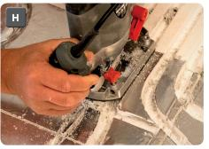
Using a router with bit set to 17mm depth gentle cut the new channel following the marker pen layout **(H)**. Ensure the channel is clear and free from debris, if required the channel can be lined with aluminium tape. Lining with aluminium tape is not required in areas with highly concentrated/close floor heating pipes.
