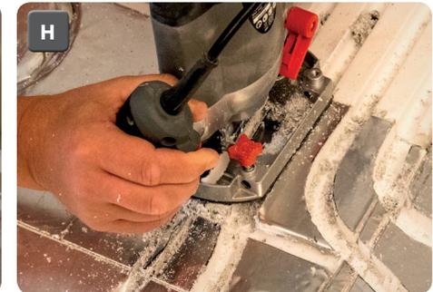
Using a router with bit set to 17mm depth gently cut the new channel following the marker pen layout (H). Ensure the channel is clear and free from debris, if required the channel can be lined with aluminium tape. Lining with aluminium tape is not required in areas with highly concentrated/close floor heating pipes.
