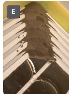
Extra pipe channels can easily be cut using a suitable router and bit. In order that a smooth bend is formed lay and shape the pipe onto the area where the channel is required, gently bending the pipe to follow a gentle curve. Once the lay of pipe has been established follow the curve with a marker pen, marking directly onto the board the route to be routed (F/G).
