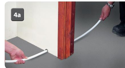
**4** When floor heating pipes need to pass through walls, drill the holes before laying and fixing boards to prevent any damage to the boards. Protect and seal the pipe ends with tape. To prevent kinking, one person should feed the pipe through the hole whilst another draws the pipe through from the other side (**4a**).
