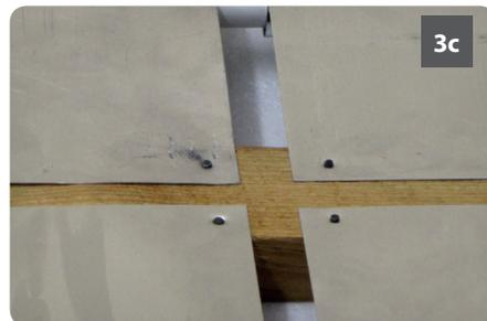
**4** Wearing safety gloves due to sharp edges lift the first spreader plate into place measuring 250mm from the wall **(4a)** and fix the spreader plate along the top of the joists using staples, nails or screws ensuring they are flush fitting **(4b/c)**. Allow a 15mm expansion gap between each plate. A good tip is to press a short length of pipe into the pipe channel to help line up the plates before fixing in place **(4d)**.
