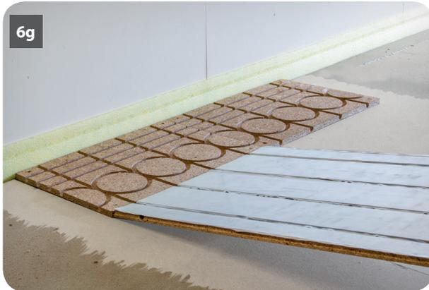
Once the first strip of end/transitional panels have been laid, apply more adhesive in a strip approximately 1250mm wide, parallel to the wall (6g), again leave adhesive to become tacky and commence laying main panels, working towards the opposite wall.
