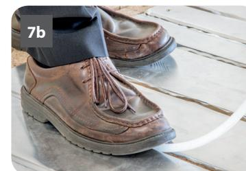
Walk the pipe into the channels in the overfloor boards ensuring the pipe is pushed securely into the bottom of each channel (7b).
