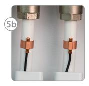
Auto balancing actuators must be wired in accordance with Wunda wiring guide. When the floor heating system is fully commissioned and thermostats call for heat, each individual actuator will activate and self-calibrate.
