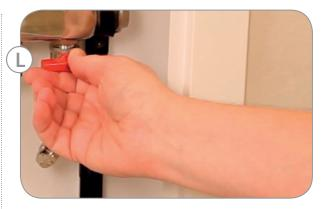
If pressure drops investigate and remedy, the mains water supply hose can be removed, leave the drain hose in place as this will be required to release the pressure at a later stage. It is good practice to leave the system under pressure whilst laying of final floor finish to indicate any possible damage to the loops of pipe.
