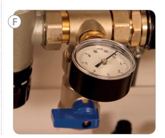
Connect the mains supply hose to the top flow bar red tap. Connect the drain off hose to the lower return bar blue tap, place the end of the drain hose into a bucket. Open both the red and blue drain taps, turn on the mains water supply to the
