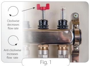
IMPORTANT: Adjust flow rate by hand only using the supplied red adjustment key. Do not force the flow gauge beyond fully open, as this will cause damage to the flow meter. Do not use pliers or grips to adjust or over tighten the flow gauges.
