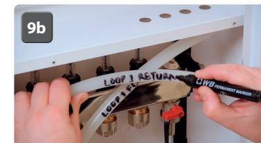
Wunda Pert/Al/Pert pipe is recommended for use in all **Overfloor** systems due to its flexible, lightweight and easy to handle properties. Always begin laying pipe at the manifold, allowing a bit extra for final connection to the manifold, identify each loop flow, return and loop number and loop length using a permanent marker **(9b)**.
