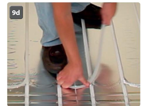
If not using a pipe decoiler the pipe can be easily installed by two people, the first walks with the pipe coil and reels it out while the second person carefully walks along the pipe pushing the pipe down into the straight pipe channel **(9c – 9d)**.
