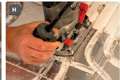
Using a router with bit set to 16/12mm depth depending on pipe, gently cut the new channel following the marker pen layout (**H**). Ensure the channel is clear and free from debris, if required the channel can be lined with aluminium tape. Lining with aluminium tape is not required in areas with highly concentrated/close floor heating pipe .
