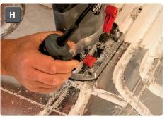
Using a router with bit set to 16/12mm depth depending on pipe, gently cut the new channel following the marker pen layout **(H)**. Ensure the channel is clear and free from debris, if required the channel can be lined with aluminium tape. Lining with aluminium tape is not required in areas with highly concentrated/close floor heating pipes.
