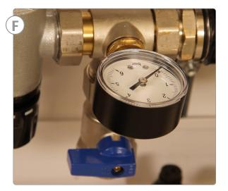
Connect the mains supply hose to the top flow bar red tap. Connect the drain off hose to the lower return bar blue tap, place the end of the drain hose into a bucket. Open both the red and blue drain taps, turn on the mains water supply to the fill hose.
