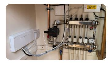
Remove all of the manual return valve caps and fit the electronic actuators in their place. Keep the manual caps for future use as they are useful if ever re-filling or purging the loops of air.
